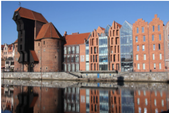
National Maritime Museum in Gdańsk. Centre for Maritime Culture (to the right) and the Crane (to the left). Photo B. Galus
