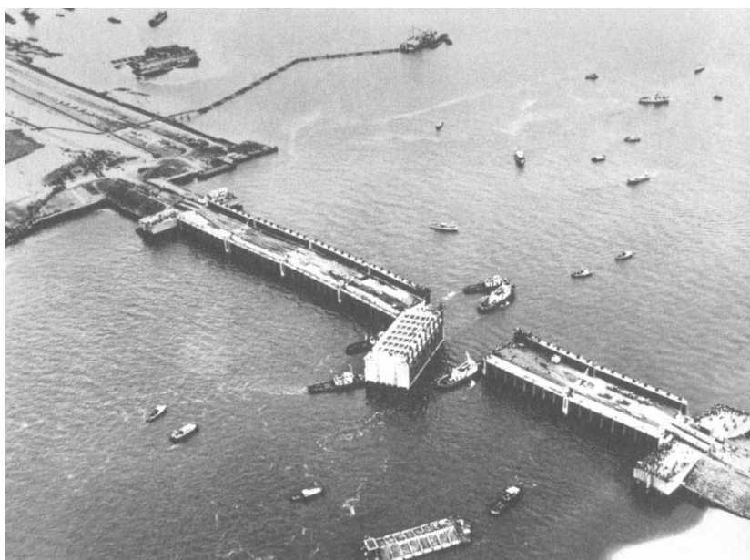
Fig. 23 The last culvert caisson to close the Veerse Gat strait April 1961. After Steenbrink 2016.
